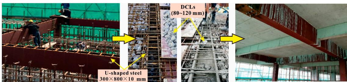
**Figure 1.** Practical application of U-shaped steel beams filled with DCLs and FC.
