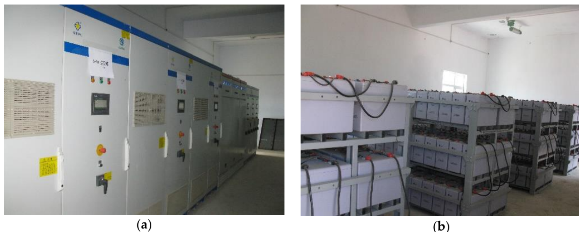
Figure 2. Equipment of PV plant: (a) PV inverters; and (b) energy storage systems.
