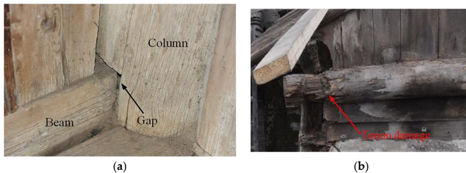
**Figure 3.** Damages of the mortise-tenon joint: (a) Gap between the mortise and tenon; (b) damage in the tenon.
