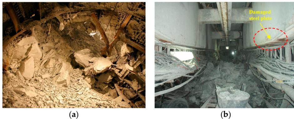
**Figure 3.** Rockburst in drainage tunnel: (a) Tunnel boring machine (TBM) is buried and (b) 80 mm steel plate is damaged.
