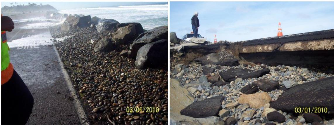
**Figure 2.** Flooding and undermining of Highway 101 in the study area during a March 2010 event. Courtesy of City of Encinitas.
