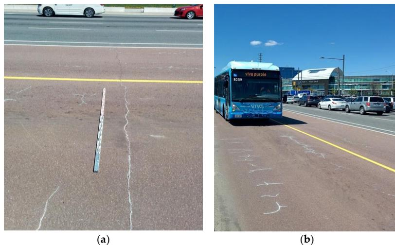
**Figure 10.** Early signs of cracks observed in sections paved with the Initial Red mixture after few years of in-service: (a) premature thermal cracking; (b) wheelpath fatigue cracking. The white colour of cracks is because of a chalk used for mapping.
