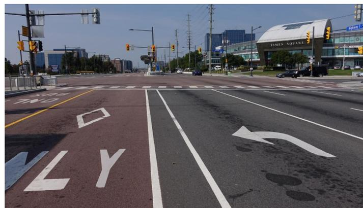
**Figure 8.** Monitored discoloration caused by oil drips and formation of oil streaks.
