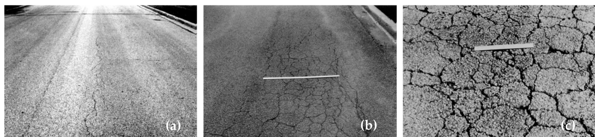
Figure 4. Distress images used in the description of alligator cracking in ASTM D 6433-11 Standard: (a) low, (b) medium, and (c) high severity levels. Reproduced with permission from [36]. Copyright 2011 ASTM.
