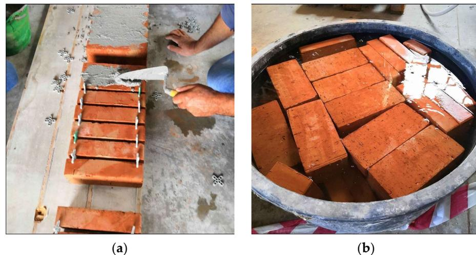
**Figure 4.** Masonry wall preparation: (a) application of the mortars and (b) bricks soaked in water.
