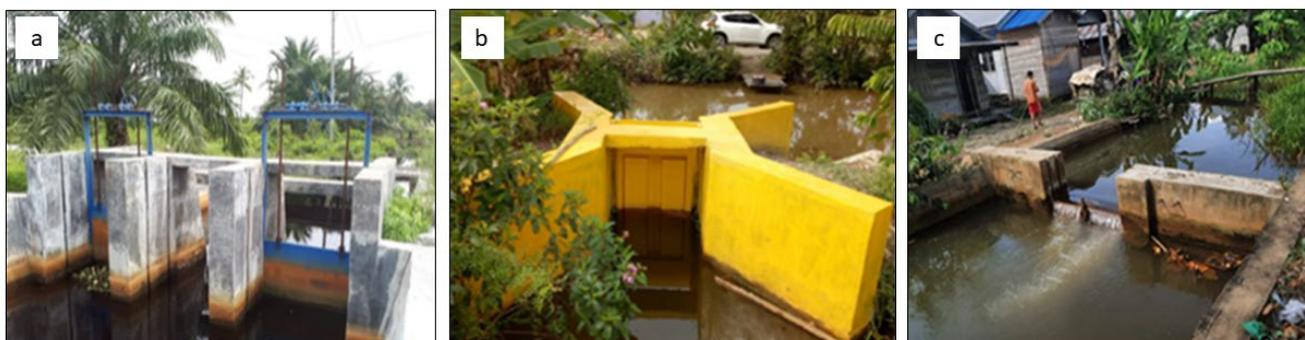
**Figure 5.** Types of water gates: (a) flapped water gate, (b) swaying water gate, (c) stoplog water gate. Photo by Author/Khairil Anwar.
