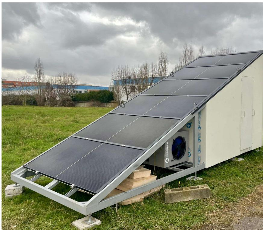
**Figure 5.** Sunthalpower: a system that integrates all the energy generation, storage, and distribution.
