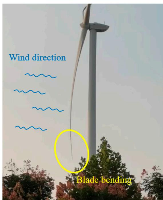
**Figure 1.** Wind turbine blade bending.
