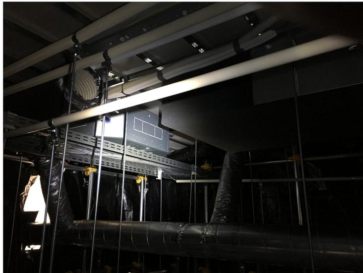
**Figure 8.** Our experiment site of the ceiling environments. The width and length was 3.5 m, and the height was 1.5 m. This site included some hanging bolts and an air conditioner and a duct pipe.
