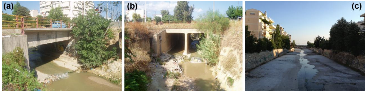
Figure 2. Typical examples of the condition of the drainage network in Athens including (a) cases of reduced cross sectional area due to bridge construction, (b) torrents covered or converted into streets and (c) buildings built directly alongside the riverbed in flood-prone areas.
