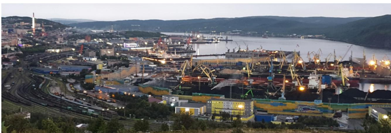
**Figure 6.** Murmansk port zone with a visible yellow-green screen offering protection from coal dust.
