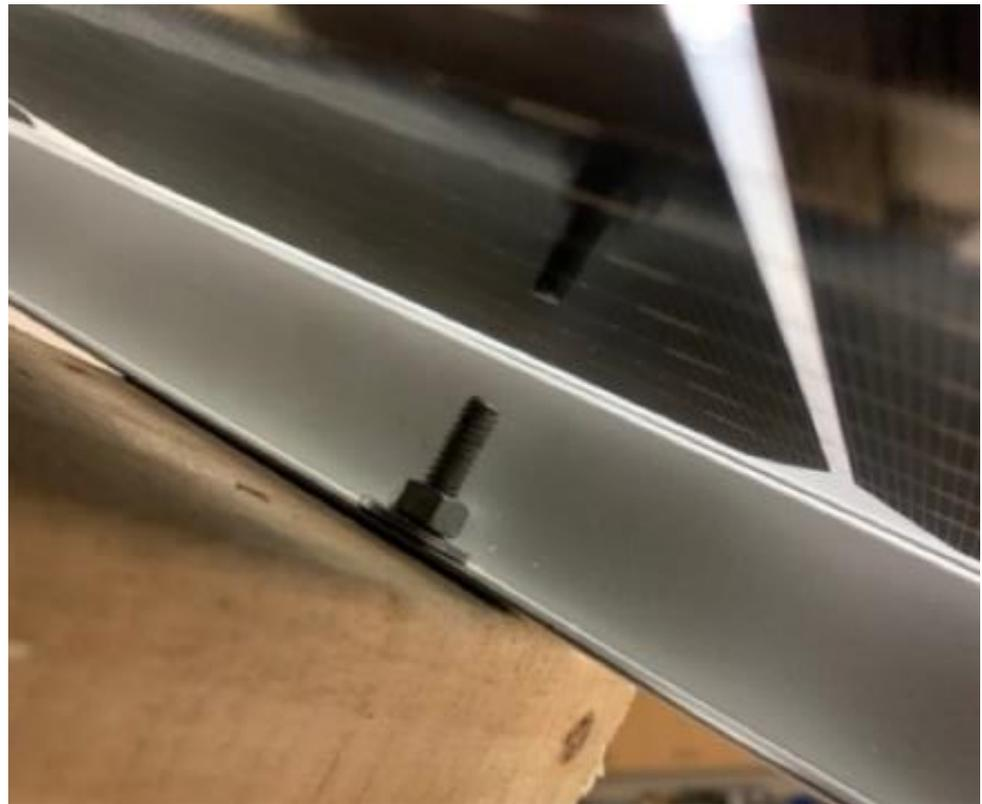
Figure 5.  $\frac{1}{4}'' \times 2\text{-}1/2''$  carriage bolt, nut, and washer used to secure the connection.
