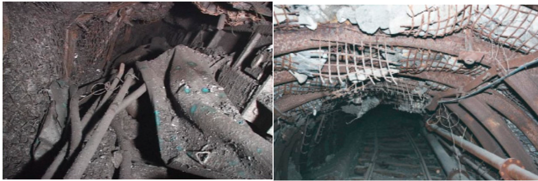
Figure 1. Field photos after severe roadway damage.
