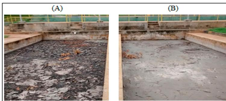
**Figure 1.** (A) Drying bed with dry primary sewage sludge. (B) Drying bed with primary sewage sludge after discharge.
