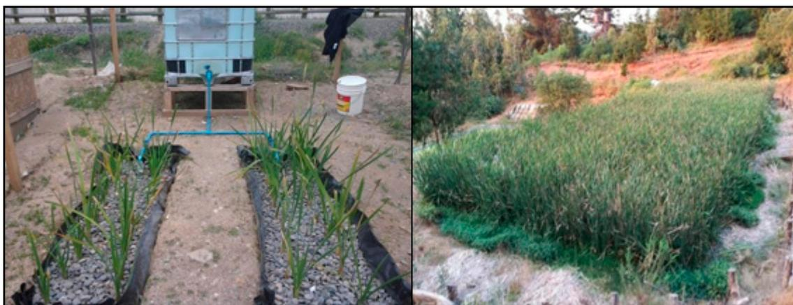
**Figure 3.** Wetlands of horizontal subsurface flow. (Left) Pilot wetlands, located in dependencies of the University of Bío Bío, Concepción. (Right) Real-scale wetland, located in the Recreational Center Ainahue, Hualqui.
