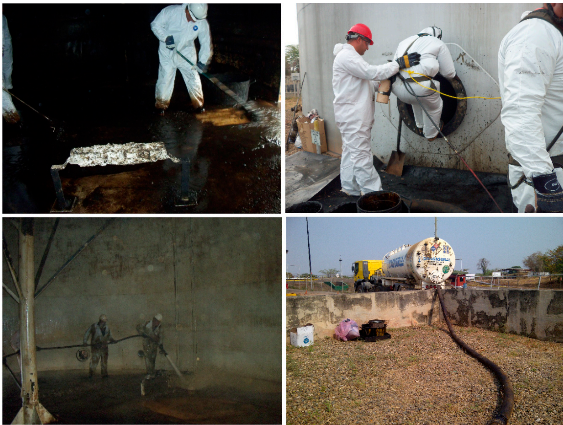
Figure 5. Manual cleaning of crude oil tank [22].
