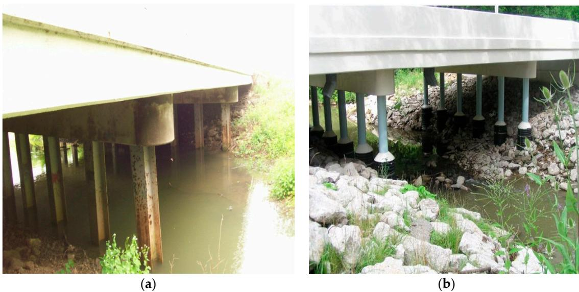
**Figure 1.** H-Pile: (a) Pier before encasement, and (b) pier after encasement (Source: ODOT).
