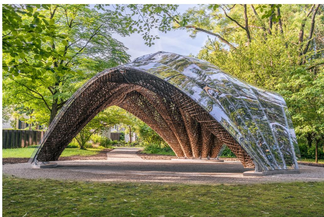
**Figure 6.** Biomimetic pavilion installed in the Botanic Garden of the University of Freiburg in 2021. The robotically manufactured flax/sisal components were inspired by the wooden cores in the trunks of various columnar cacti and prickly pears (reprinted with permission from © ICD/ITKE/IntCDC University of Stuttgart, Rob Faulkner).
