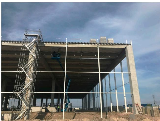
**Figure 1.** Load-bearing structure for a single-story warehouse on a site with severe seismic action, ground acceleration  $a_g = 0.35$  g. Reproduced with permission from ©SDC Project [[https://www.sdcproject.ro/wp-content/uploads/2018/10/IMG\\_1887-08-06-18-11-30-1.jpg](https://www.sdcproject.ro/wp-content/uploads/2018/10/IMG_1887-08-06-18-11-30-1.jpg) (accessed on 4 March 2024)].
