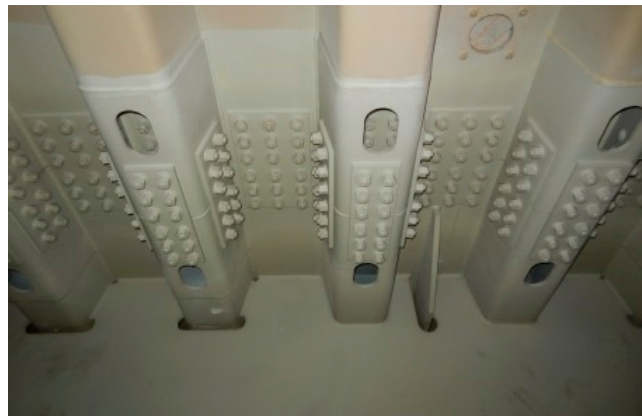
Figure 1. The bolted splicing part in the box girder of a bridge.
