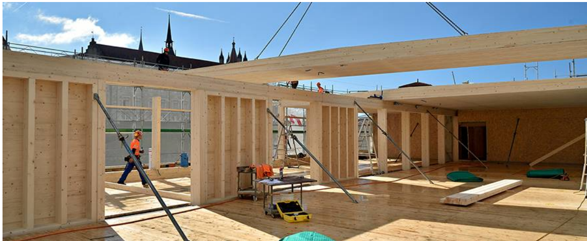
Figure 8. On-site assembly of the prefabricated wooden elements.
