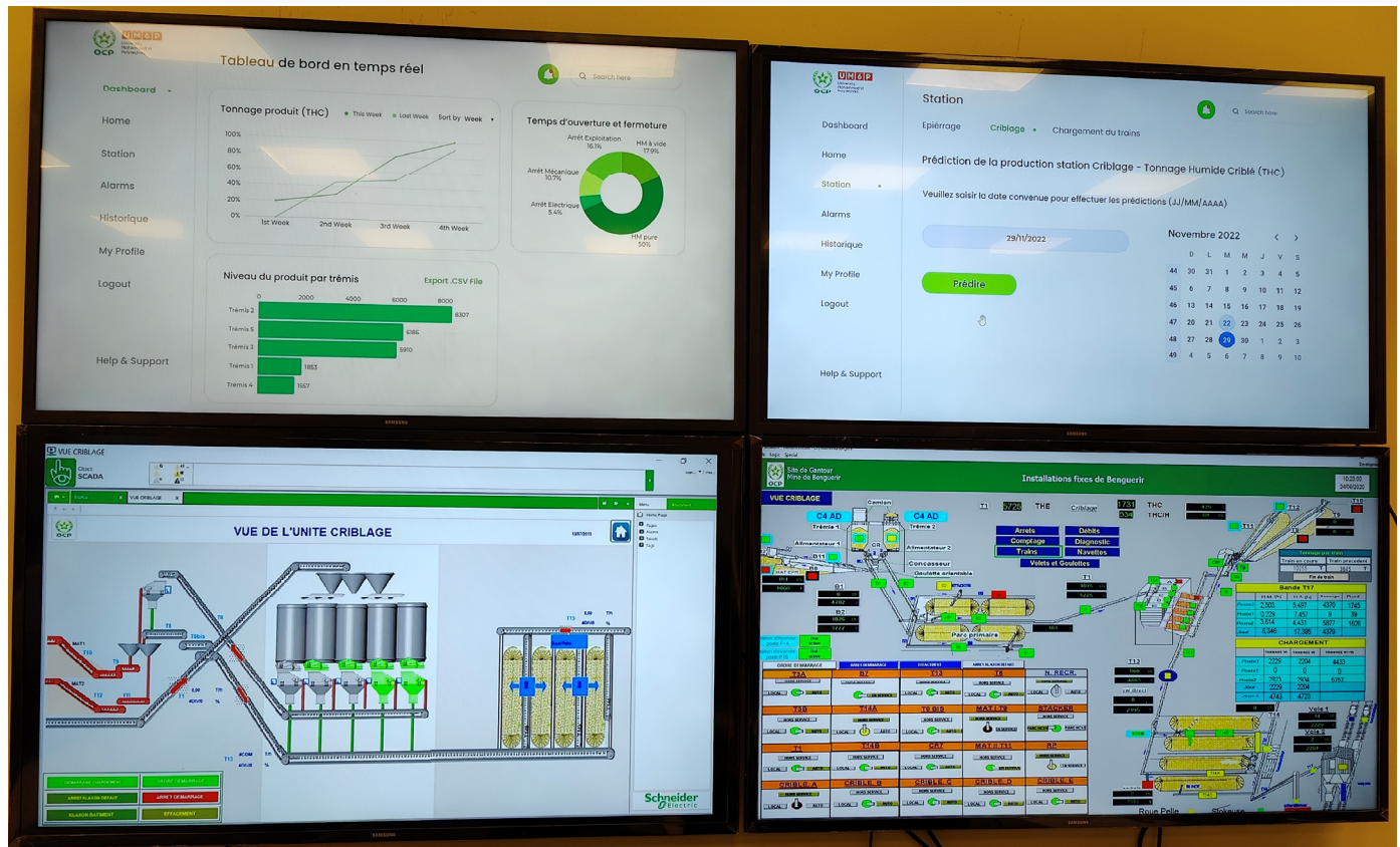
Figure 12. Integration of production management system (PMS) in the control room combined with SCADA monitoring of screening station.
