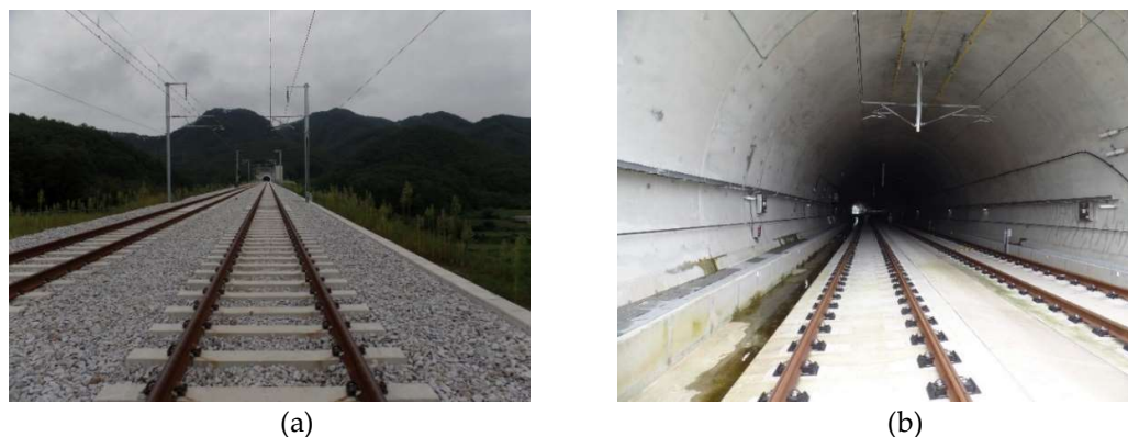
Figure 4. Dynamic response trackside measurement sites (ballasted and ballast-less slab); (a) ballasted track; (b) ballast-less slab track.
