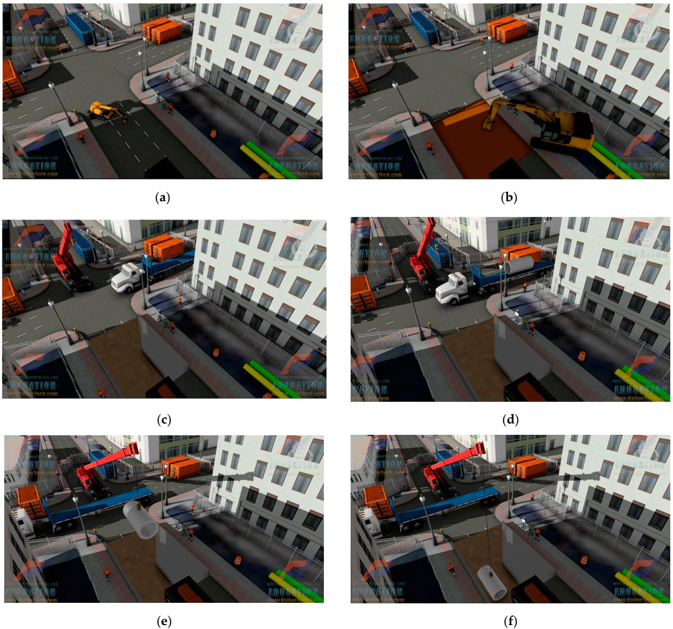
**Figure 8.** Four-dimensional simulation of MUT construction using C&C in Fuzor 2022 software: (a) demolition of the pavement; (b) trench excavation; (c) installation of trench shoring system; (d) delivering a section to the site; and (e,f) lowering the tunnel section.
