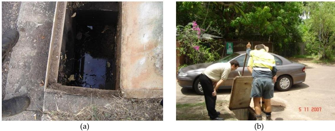
**Figure 1.** (a) Drain sump with dry season stagnant water in Rapid Creek; (b) inspecting drain pits.
