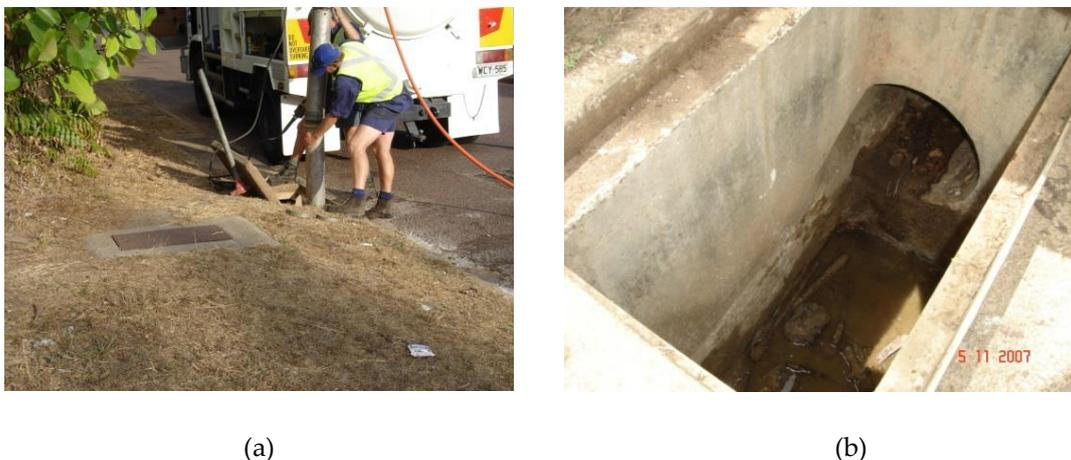
**Figure 3.** (a) Sump being cleaned by jet/vacuum; (b) cleaned sump ready for concrete filling.
