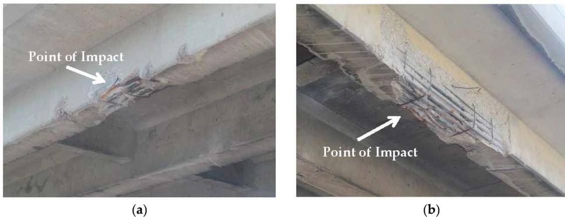
**Figure 3.** Impact damaged reinforced concrete (RC) girders (a) Impact side of Girder G1; (b) Back side of Girder G4.
