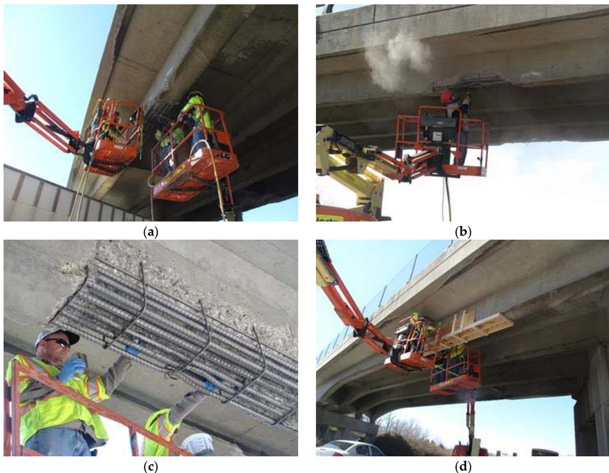
**Figure 9.** Concrete repair of RC girders (a) Remove loose concrete; (b) Grit blasting steel rebar; (c) Application of primer coating on rebar; (d) Setting up formwork for repair mortar.
