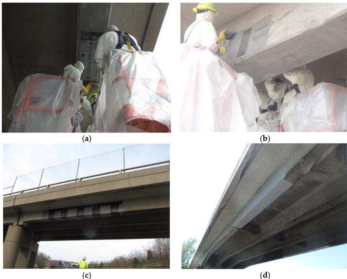
**Figure 10.** CFRP Strengthening (a) CRP applied to bottom surface; (b) Covering CRP on sides; (c) CFRP U-wraps and anchor strips applied over CRPs; (d) Ultraviolet (UV) protective coating applied over retrofit.
