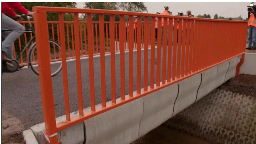
**Figure 10.** 3D printed bicycle bridge developed by Eindhoven University of Technology (Reproduced from [52]).
