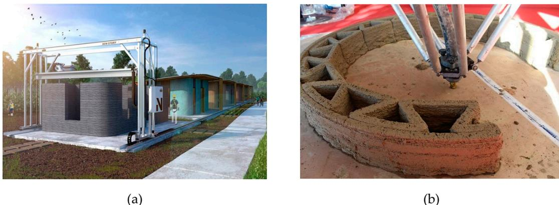
**Figure 4.** (a) ICON Vulcan II (Reproduced from [23]) and (b) WASP Crane apparatus (Reproduced from [24]).
