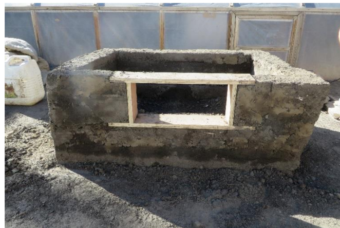
Figure 3. Detail of wooden frame for solar cooker drawer.
