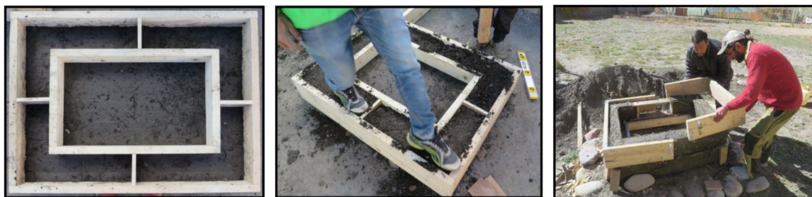
Figure 4. Timber frames to standardize cooker structure and assure reliable quality ( left ), rammed earth construction process ( mid ), removal of frame after mud has dried ( right ).
