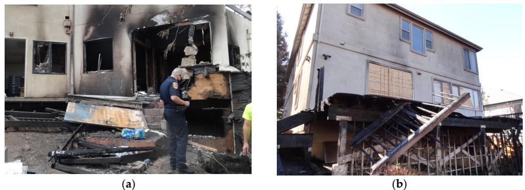
**Figure 1.** Examples of burning decks causing damage to the main structure of (a) a commercial wine-tasting room in Napa Valley and (b) a residential structure in Santa Rosa, California, during the 2020 Glass Fire. (Images taken during IBHS’s post-event investigation).
