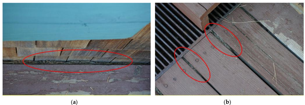
**Figure 10.** (a) Deck to wall connection, with accumulation of vegetative debris in gap between deck and vertical wall. (b) Debris accumulation in the gap between deck boards [4].
