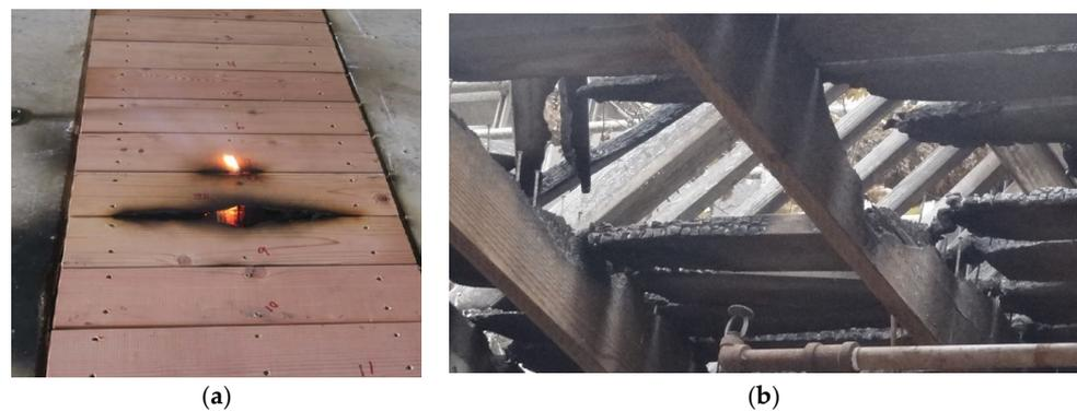
**Figure 11.** (a) Fire propagation along the joist towards the test building (b) Fire propagation along the joist towards the main building in a commercial wine-tasting room in Napa Valley, California, during the 2020 Glass Fire. (Images taken during IBHS's post-event investigation).
