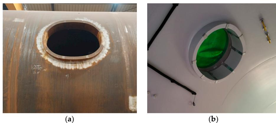
**Figure 2.** Photos of typical ventilation openings: (a) during fabrication; (b) finished (courtesy of Ateş Wind Power).
