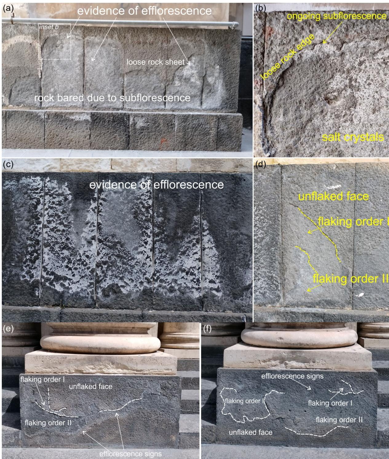
**Figure 4.** Efflorescence phenomenon and subflorescence effects observed at the igneous rocks employed as cladding along the lower part of the north-facing façade (a,b), STW (c,d), and as column II and III stereobates along the south-facing prospect of the building (e,f).
