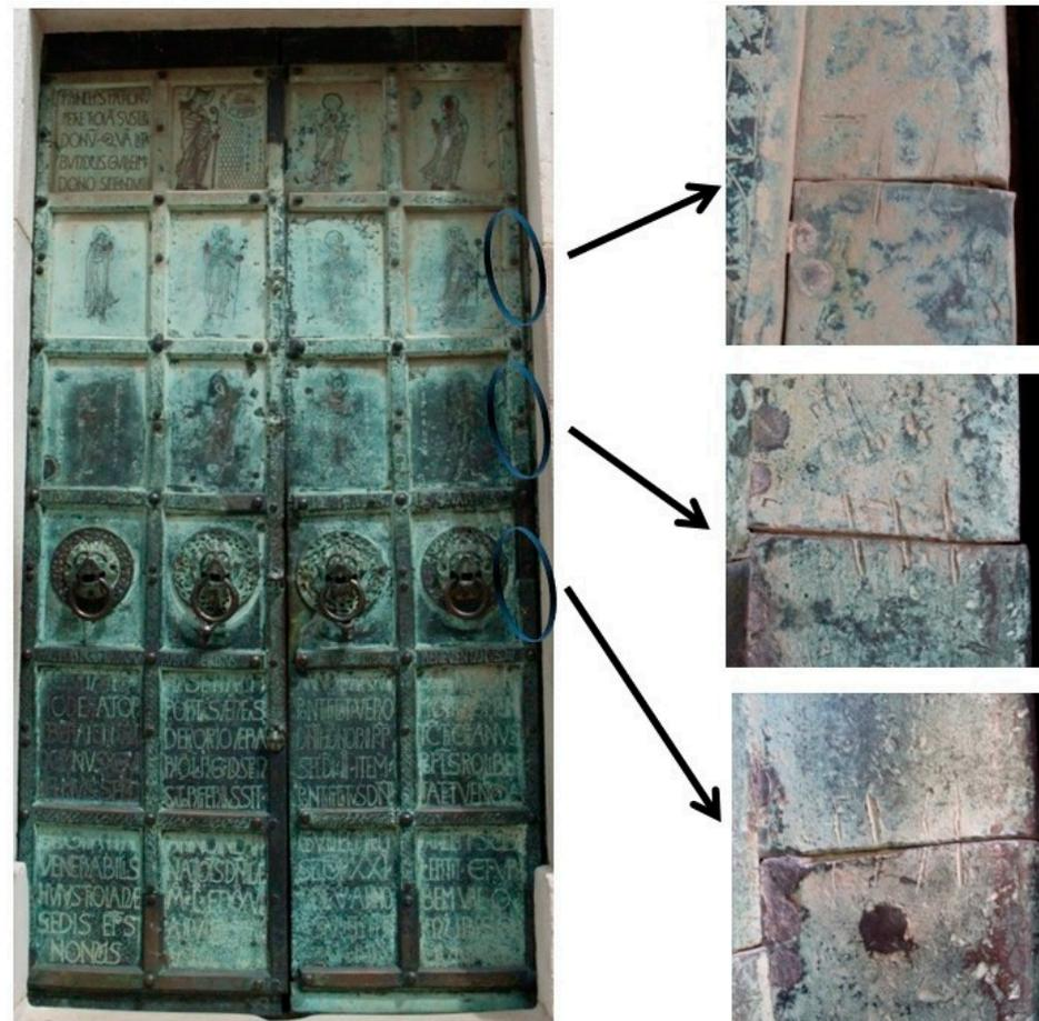
**Figure 6.** Picture of three complementary engravings between two neighbouring panels, inscribed to facilitate the assembly of the door.
