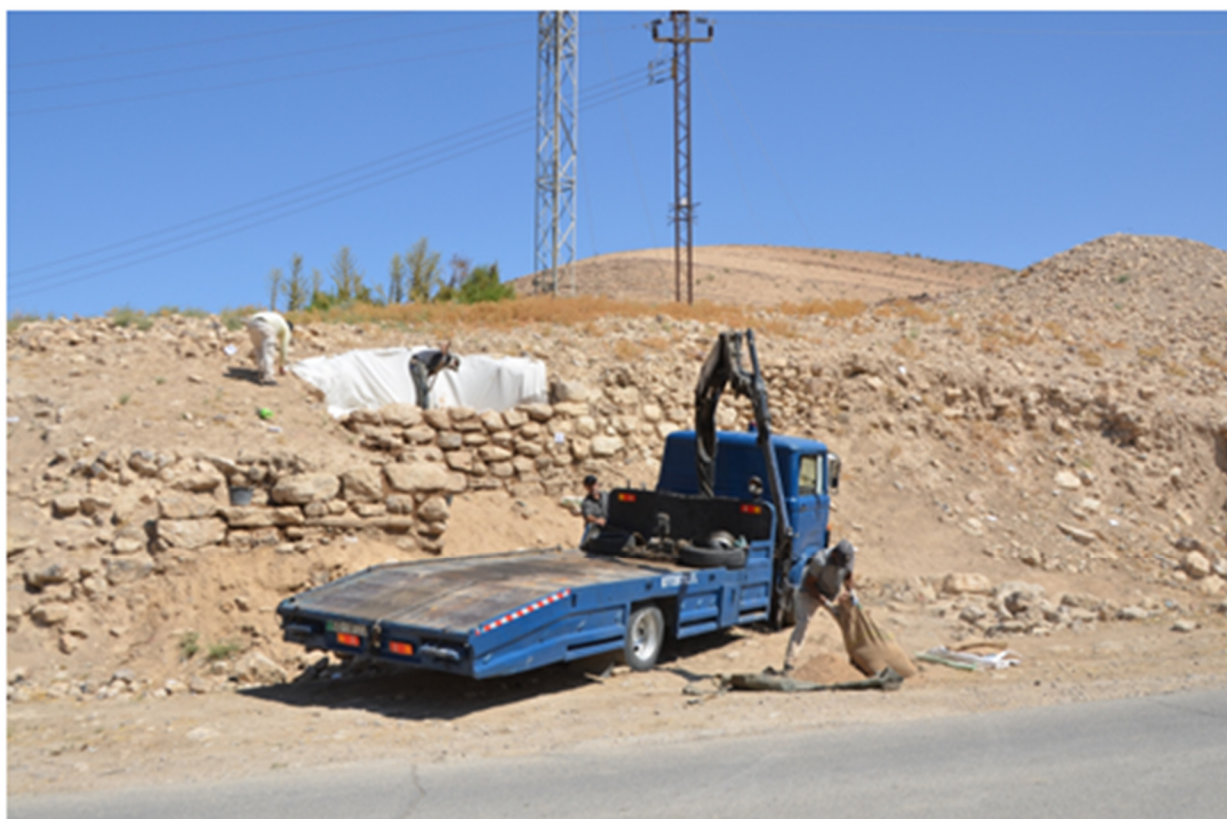
Figure 23. Khirbat Iskandar, KI-RC02: fabric inside the restored wall to separate the original from the restored parts, to stabilize the inside, and regulate water drainage, in July 2023 (photos by Khaled Al Wekhean, © Archaeological Expedition to Khirbat Iskandar).
