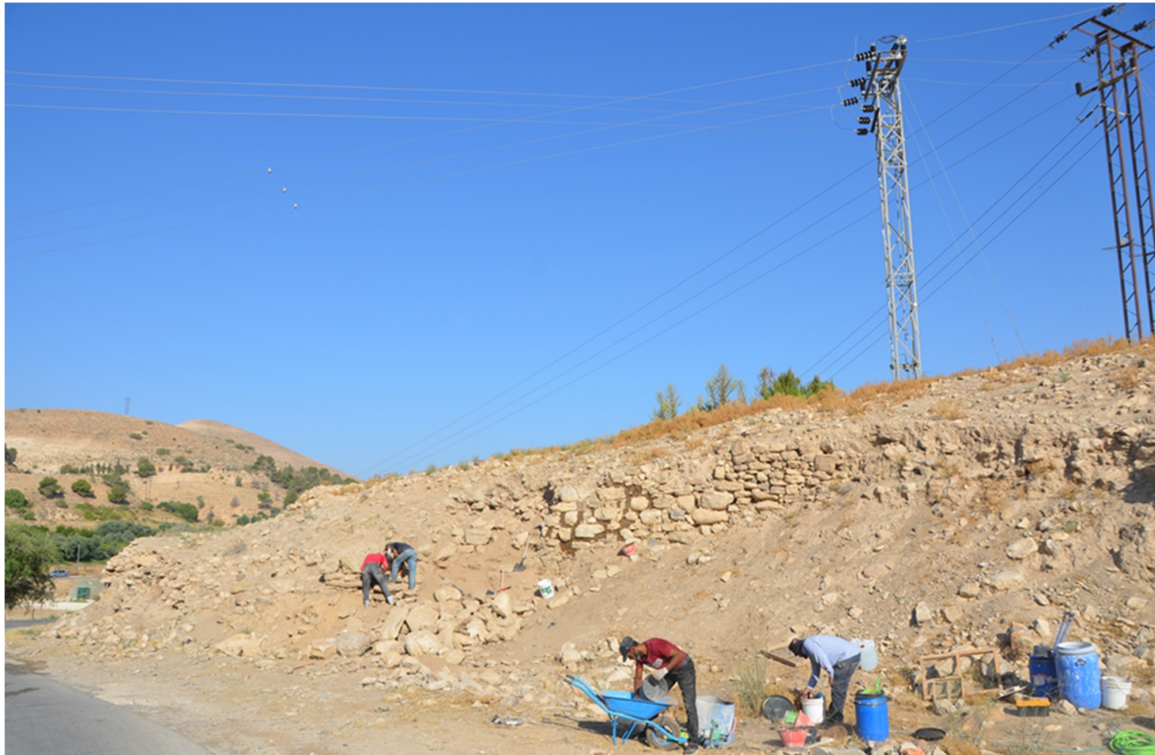
Figure 18. Khirbat Iskandar, KI-RC02: the application of the rough earthen coating on the restored façade of the collapsed walls, looking toward the south-west, in July 2023 (photo by Khaled Al Wekhean, © Archaeological Expedition to Khirbat Iskandar).
