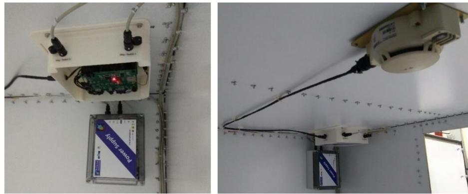
**Figure 12.** The INTELLICONT devices and the smoke detector installed inside the container.
