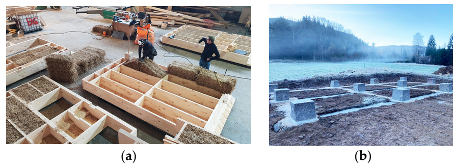
Figure 2. (a) Detail of the assembly of the wooden structural frame; each element is filled with straw. (b) A picture of the granite blocks and the concrete trusses that constitute the foundations (Source: studiolada.fr (accessed on 15 April 2023)).
