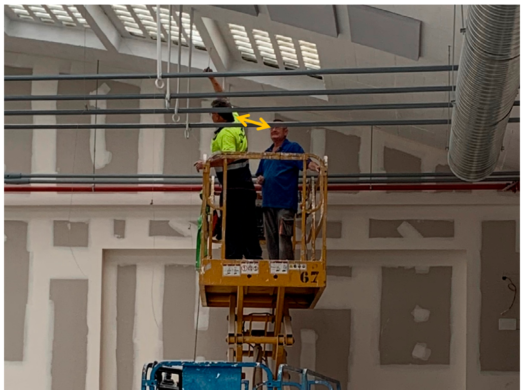
Figure 4. Workers installing false ceiling supports on a lifting platform. The photograph marks the distance between the workers, which is lower than 1.00 m (author's photograph).
