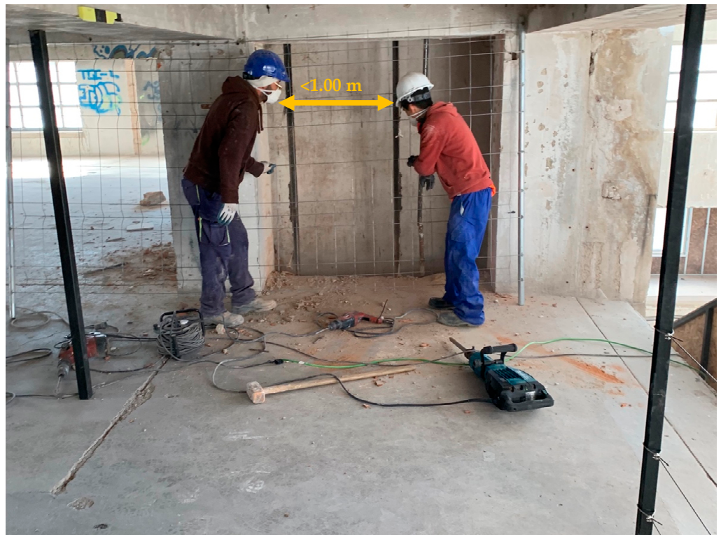
Figure 3. Workers exchanging a protection element in an elevator shaft in a building's interior rehabilitation work. The photograph indicates the separation distance between workers (author's photograph).
