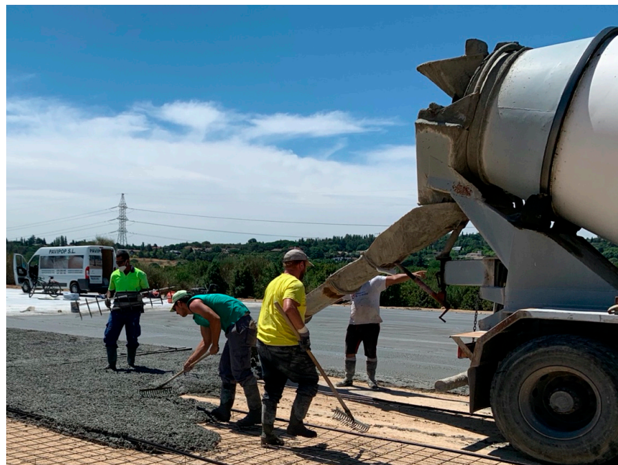
Figure 2. Workers spreading concrete on an open-air screed without keeping safety distance (author's photograph).
