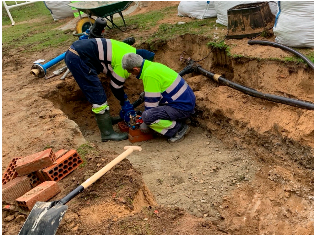
Figure 1. Workers finishing hydraulic pump placement in civil work for water conduction. The work had to be performed in pairs without a safe distance (author's photograph).
