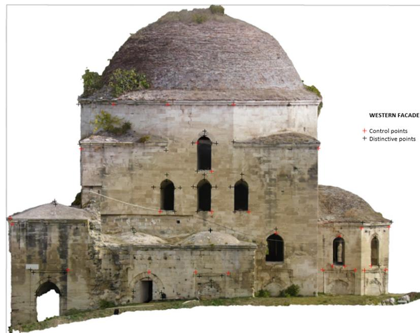
**Figure 29.** Error estimation for the western facade orthophoto derived from photogrammetric processing.
