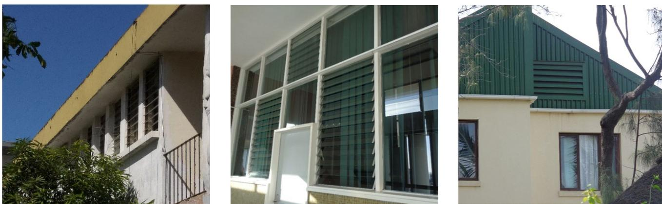
**Figure 8.** Example of ventilation using adjustable vents in windows to promote evaporative cooling. In addition, ventilation through the chimney effect with an air inlet at the bottom and outlet at the top of the roof (Beira, Mozambique).
