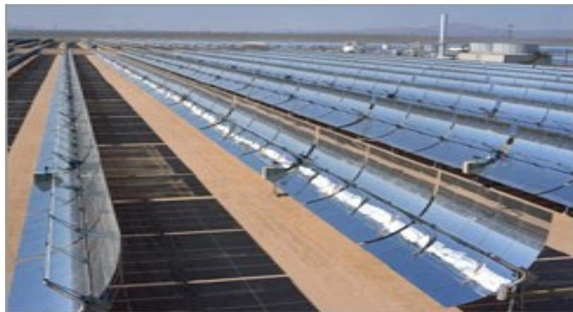
**Figure 6.** Parabolic Collector of the Power Plant.
