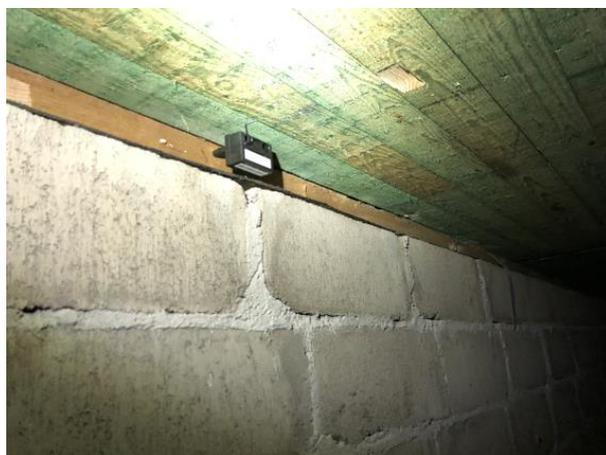
**Figure 2.** Crawlspace interior. The picture shows the concrete block wall, the treated wood sill plate on the wall (brown/green), and the treated wood ceiling (light green). A black humidity logger is placed on the sill plate, and two rectangular sampling sites are visible, one on the sill plate (far left) and one on the ceiling (middle).
