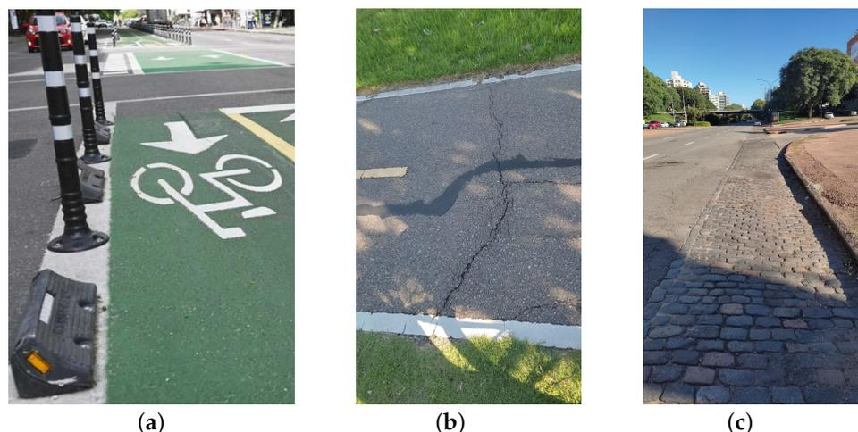
**Figure 5.** Examples of different pavement maintenance conditions within the cycling infrastructure of Montevideo (own photographs). (a) Bicycle path with good quality pavement (location: 18 de Julio). (b) Bicycle path with deteriorated pavement (location: Avenida Italia). (c) Street with poor conditions for cycling (location: Bulevar Artigas).
