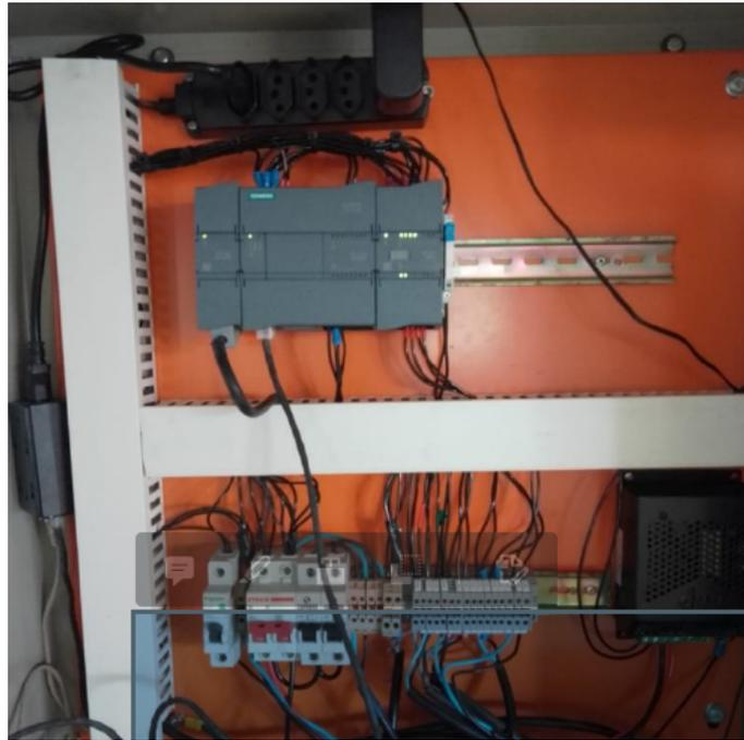
**Figure 13.** Control panel with Siemens controller. Source: Google Maps.
