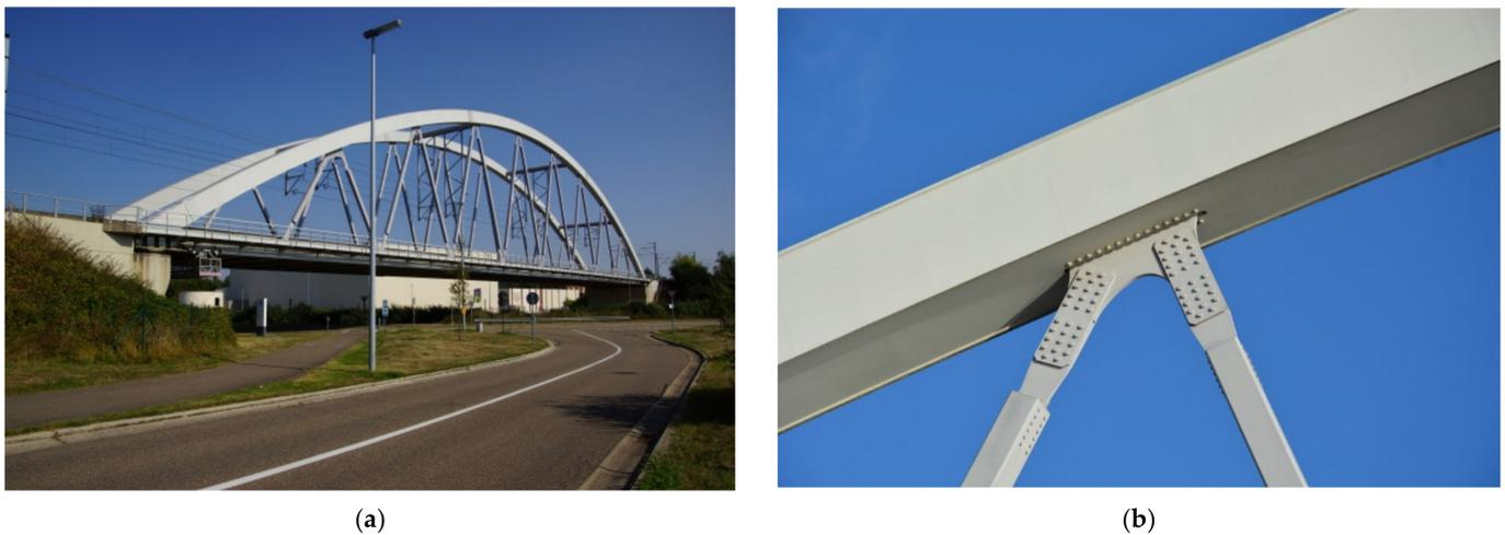
**Figure 3.** (a) The KW51 bridge in Leuven and (b) Example of bolted connection between a brace and the arch of the bridge (Reprinted from ref. [54]).
