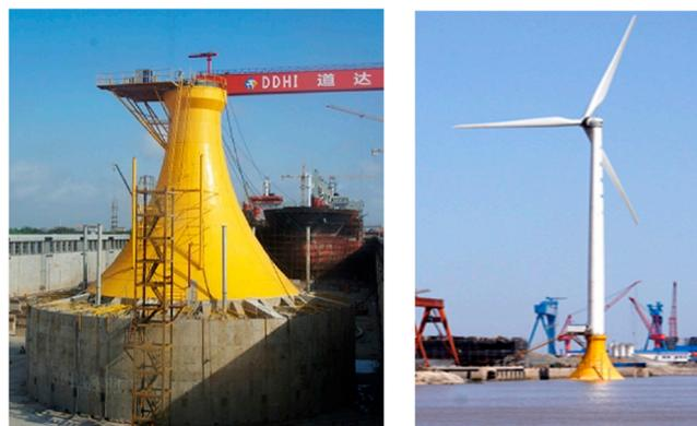
**Figure 1.** Composite bucket foundation (CBF) with concrete skirt of 2.5 MW in Qidong, Jiangsu Province, China.
