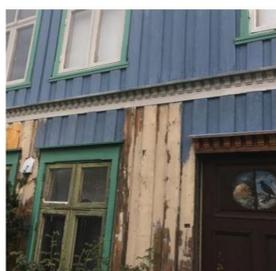
Figure 5. Deteriorating façade (NTNU).
