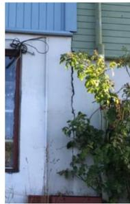
**Figure 10.** Crack between the buildings Strandveien 19 and 21 (NTNU).
