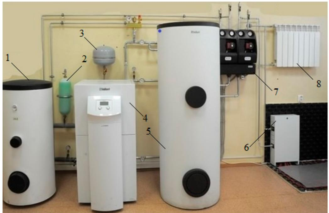
**Figure 1.** Research heat pump plant. 1—cold water tank, 2—expansion tank, 3—membrane tank, 4—heat pump, 5—hot water tank, 6—distribution manifold for underfloor heating, 7—pumps and water collector, 8—heating radiator.
