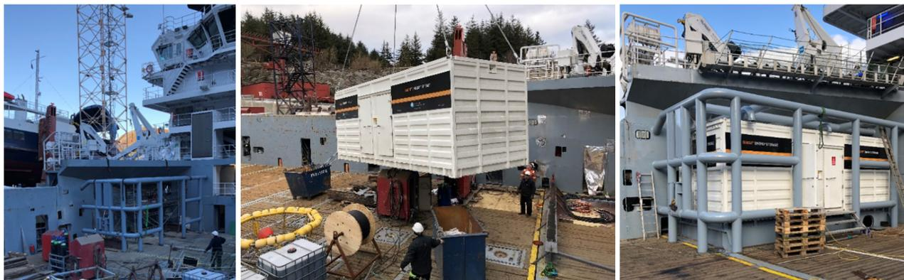
**Figure 3.** The installation of one unit of a 630 kWh BESS on a OSV in March 2018.
